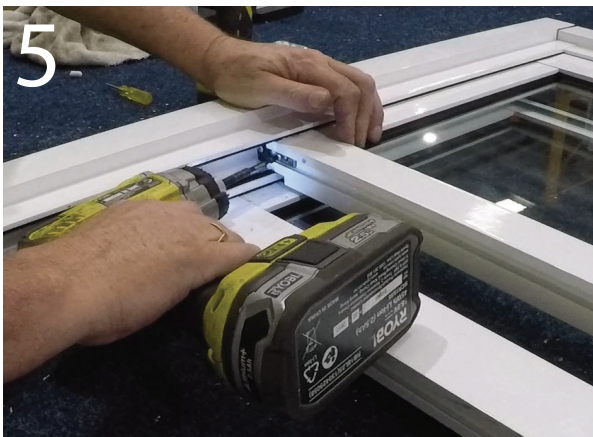
5. Screw/pop-rivet friction feet onto bottom of sash
