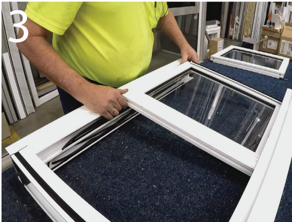
3. Install sash(es) into frame
