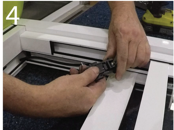
4. Fit friction foot onto end of spring after removing cord and slide up into the side of the sash
